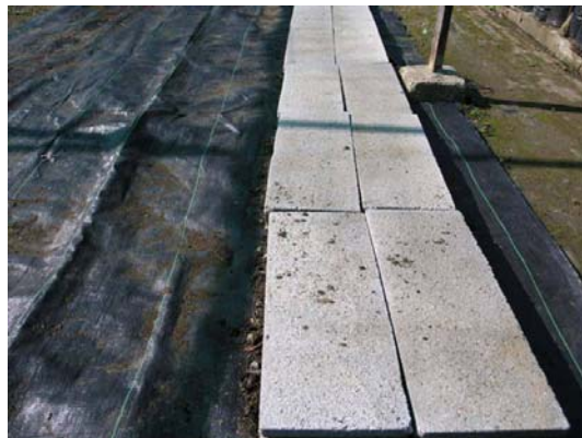
Figure 17. Platform for placing the bags.
